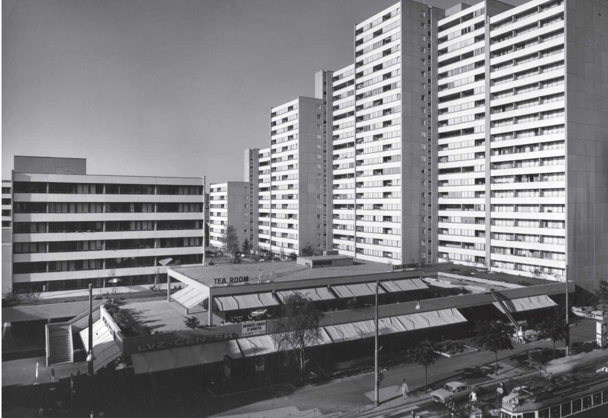
Figure 4.3 Lochergut in Zurich, where Jephtas lived in a flat formerly the home of the writer Max Frisch. Source: Baugeschichtliches Archiv der Stadt Zürich, BAZ_160347.
